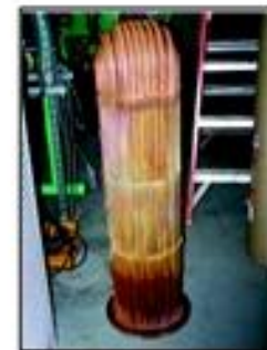
Heater coils after being cleaned with Dynamic Descaler®.
